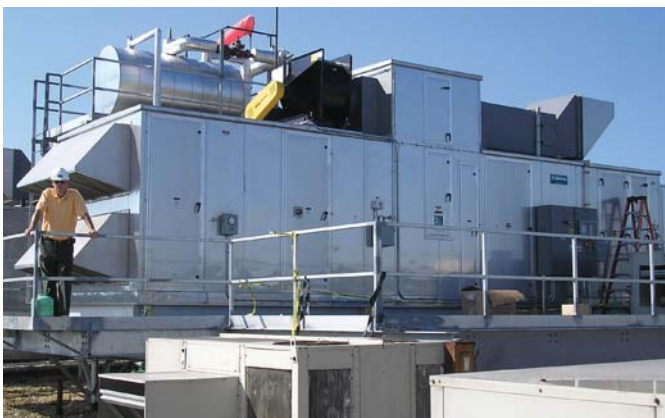
Munters Condensation Control System equipped with PowerPurge™ installed at the Siler City, North Carolina plant.
